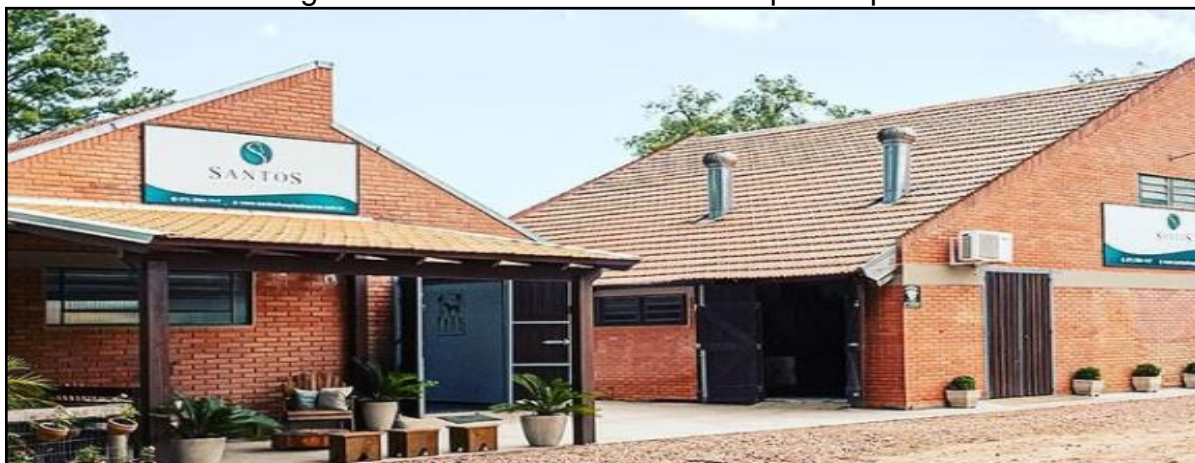
Figura 1 – Fachada do Santos Hospital Equino
