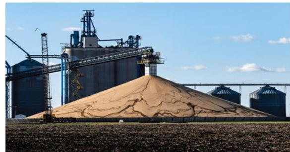
Fig. 1. Example of a stockpile.
